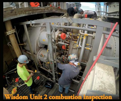
**Above** Contractors remove piping late September on Wisdom Unit 2 as part of a routine inspection. A combustion inspection is customary after a unit reaches it's 600 start up which Wisdom Unit 2 reached late this summer.
